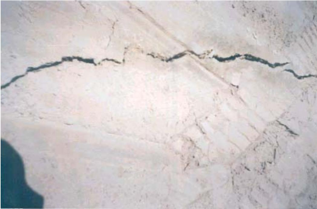
Long crack near the edge of the stack
